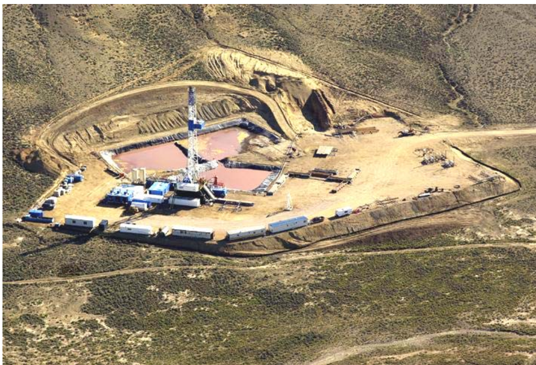
Figure 1. Drilling pad in Sublette County (photo by Ecoflight courtesy of SkyTruth). Sources of \text{NO}_x include the diesel-fired drill rig engine, which operates the drill itself, as well as pumps and generators associated with hydraulic fracturing operations, and heavy truck traffic to and from the drilling pad.
