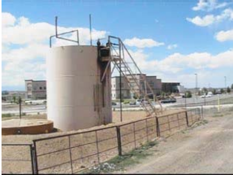
Figure 3. Condensate tanks, which store volatile liquid petroleum produced with natural gas, can be a significant source of VOCs. Emissions are invisible to the naked eye, but can be observed with the use of infrared technology. The picture above is a condensate tank in Weld County, Colorado. Below is the same tank with VOC emissions visible through an infrared camera (images from video prepared by the U.S. Environmental Protection Agency).
